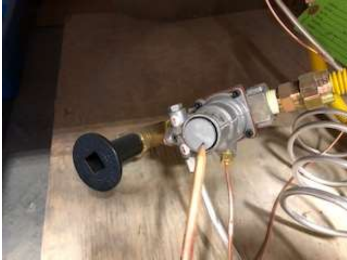
Flame Supervision Valve H15 button (grey in color). Note the pattern on the back of button for reinstallation
